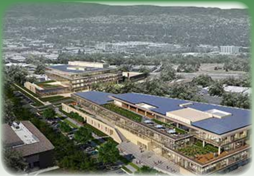
Intuit headquarters campus, Mountain View, California
